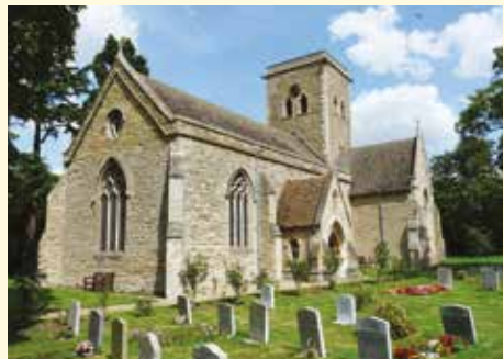
St. Mary, Bletsoe: Chancel Restoration
