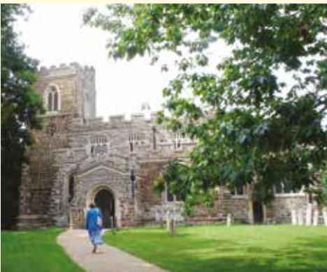
St. Nicholas, Tingritb: Masonry Repairs
