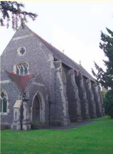
Al Saints, Long Marston: Drainage & Stonework Repairs
